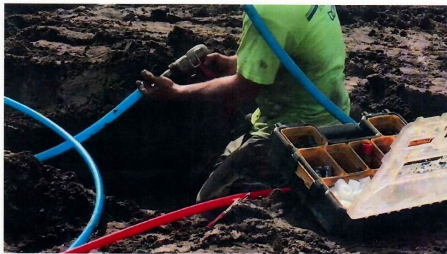
PEX being put into the ground for a geothermal HVAC system
